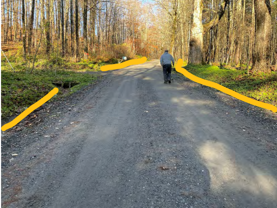
1842 before 2 heading uphill - stone line ditching both sides
