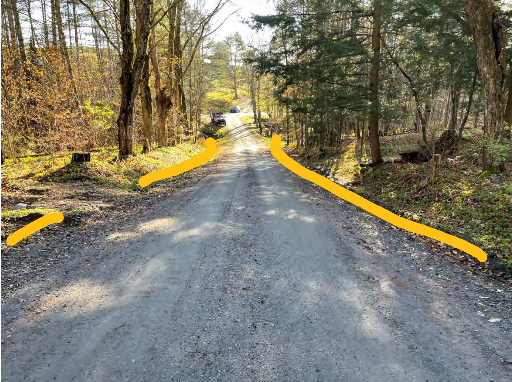
1831 before 1 – stone line ditching both sides
