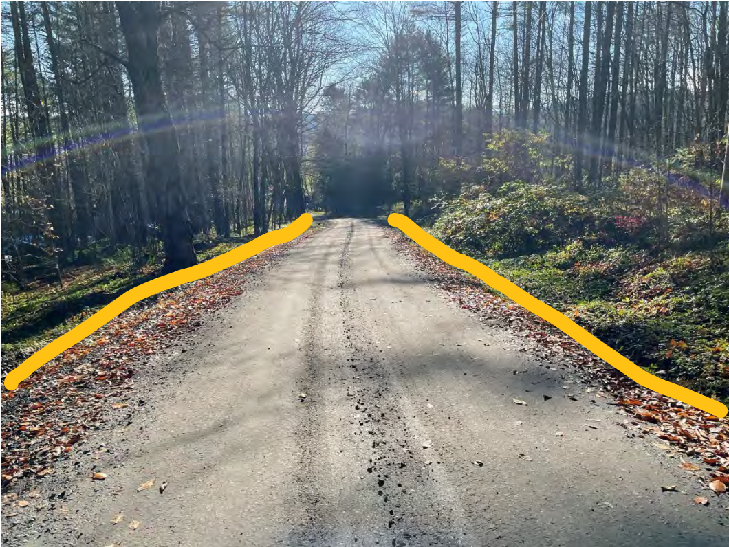
1842 before 1 - stone line ditching both sides, replace existing culverts to 18"
