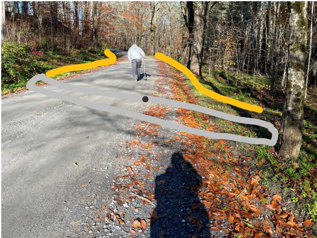
1842 before 3 - stone line ditching both sides, add back 18" cross culvert
